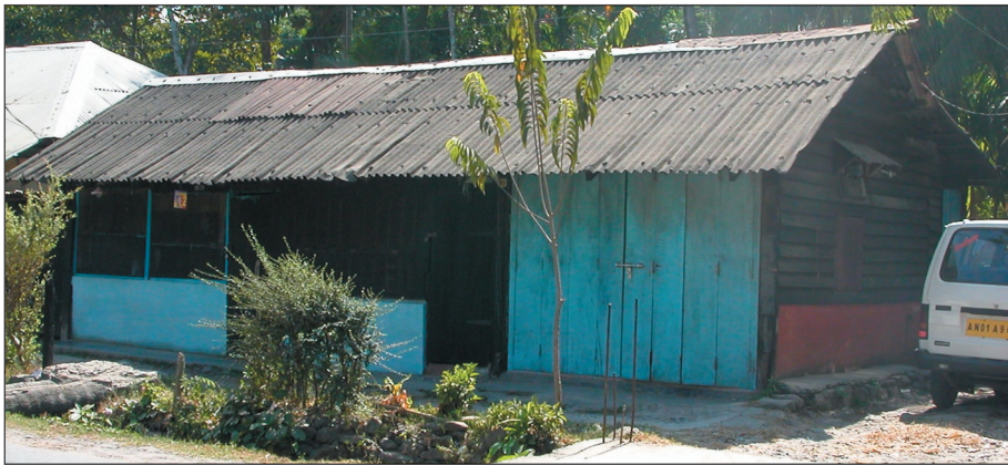
Figure 5a. Single-story wood house in Port Blair with light roof had no damage (photo: C.V.R. Murty).
