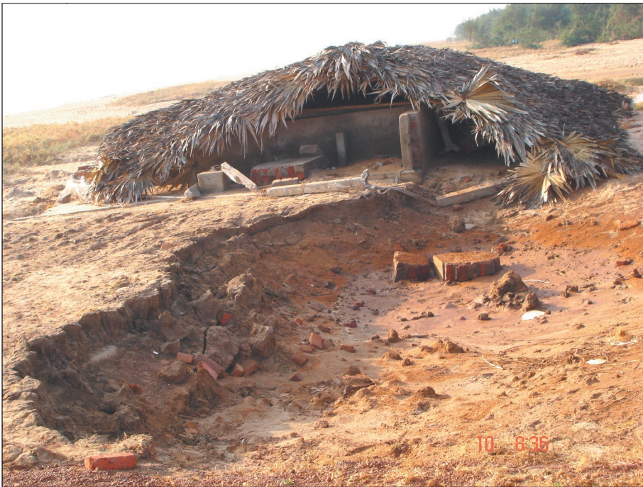
Figure 15. Mud house with thatch roof built within 100 meters of the sea at Pakala Beach in Andhra Pradesh (photo: Arvind Jaiswal).
