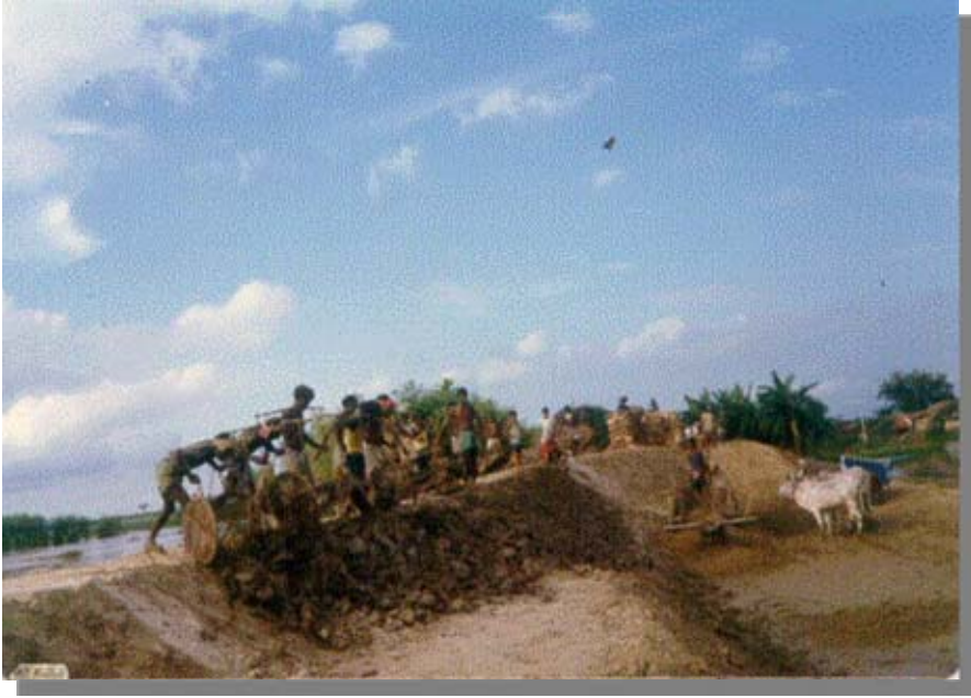
Figure 2: Restoration of a subsided embankment without any compaction
