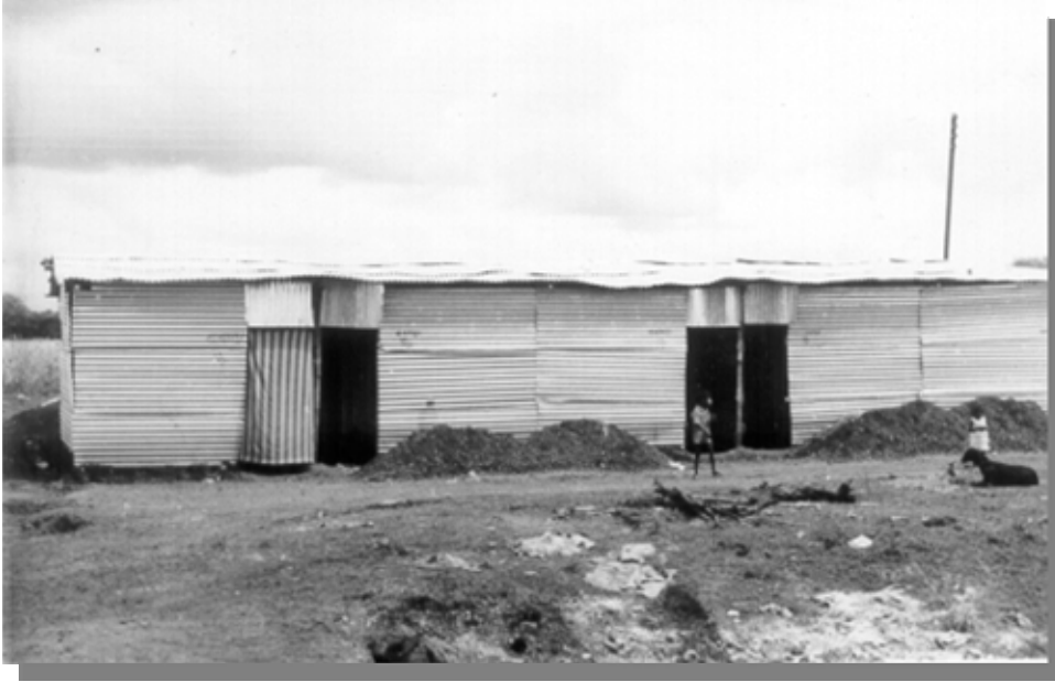
Figure 9: Temporary shelters of galvanized iron sheet were rapidly erected. Each provides shelter for five families
