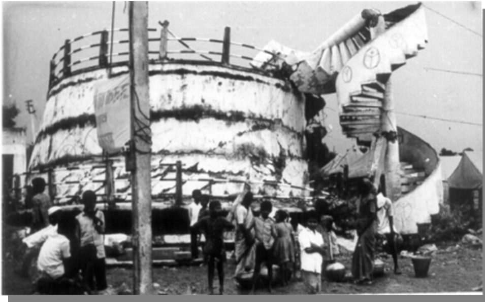
Figure 6: While most elevated water tanks performed well, this tank of Kautha collapsed straight down into its crumpled supports. Circumferential displacement of about 0.5m suggests that rotational vibration led to its collapse.
