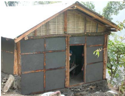
Figure 2: Traditional construction in Sikkim: (a) Typical Ikra structure (School building at Nandok in East Sikkim); (b) Ikra house under construction near Nandok; and (c) internal view (note use of wooden trusses and GI sheets in roof construction).
