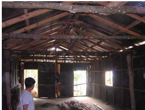
Figure 2: Traditional construction in Sikkim: (a) Typical Ikra structure (School building at Nandok in East Sikkim); (b) Ikra house under construction near Nandok; and (c) internal view (note use of wooden trusses and GI sheets in roof construction).
