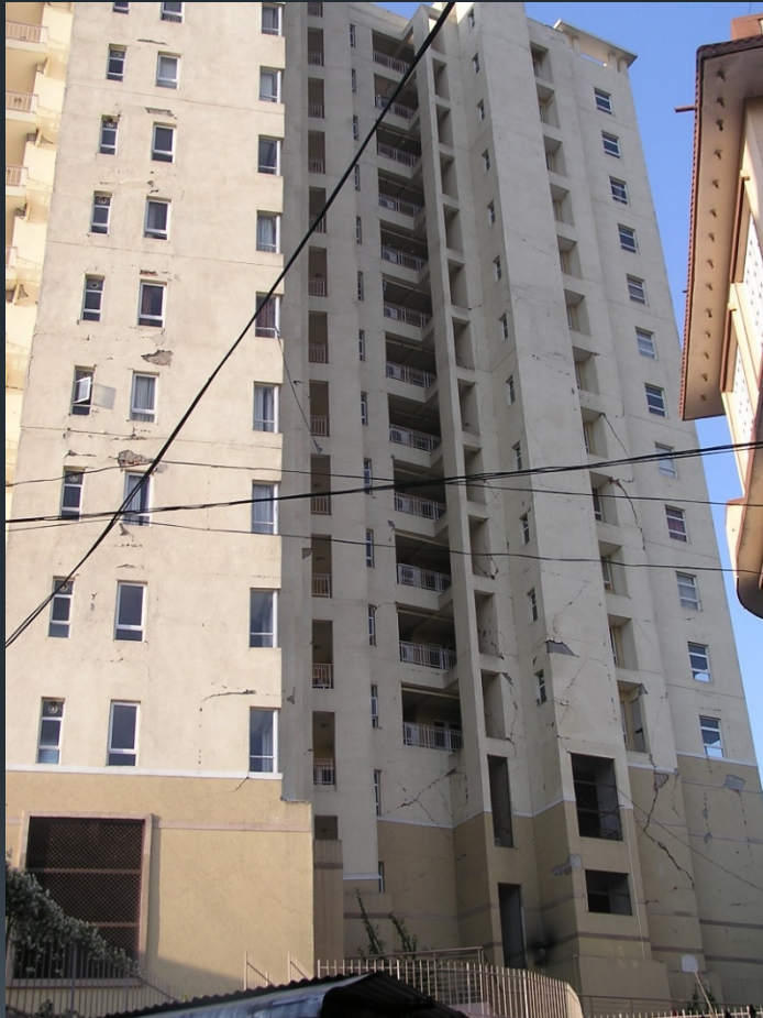
Separation of infill for boundary frames
