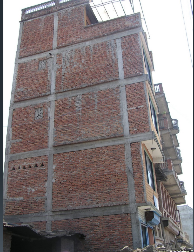
Box type construction: Extension of wall beyond column line
