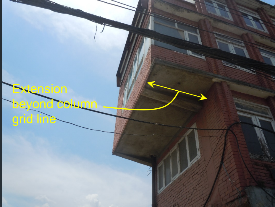
Box type construction: Extension of wall beyond column line
