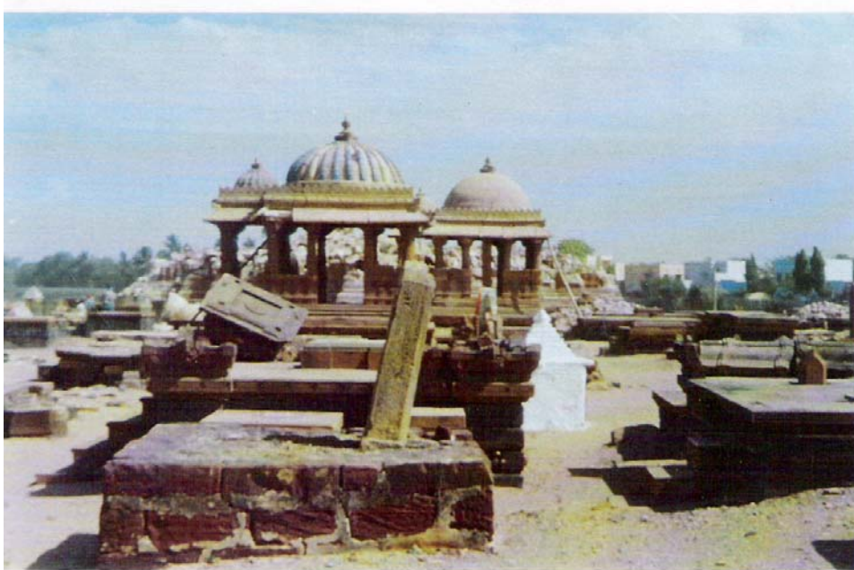
Figure 9.1 Overturned and tilted rigid objects observed at Bhuj subsequent to the 2001 Gujarat earthquake. Based on such observations one could estimate a lower bound on peak ground acceleration that might have occurred during the earthquake.
