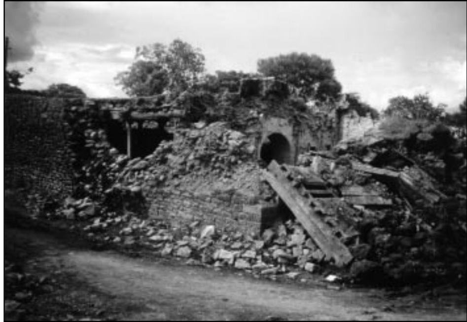
Figure 2 A typical stone masonry and mud mortar building in complete ruins after the earthquake.
