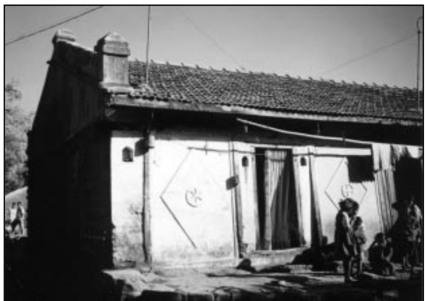
Figure 6 A typical house with a sloped timber roof covered in clay tile in the high rainfall area of Maharashtra.
