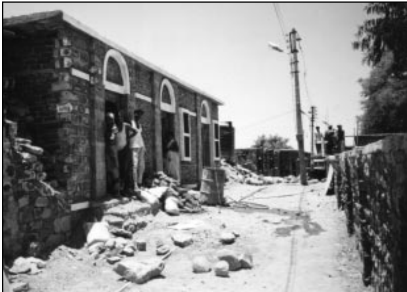
Figure 7 Tembhi village, rebuilt by HUDCO (Housing and Urban Development Corporation, Ltd., a GOI undertaking) with financial support from the German government. It is an exemplary example of donor-managed rebuilding, with an emphasis on stone masonry and cement mortar and traditional architectural detailing. Seventy-two houses were rebuilt in three years in Tembhi village.
