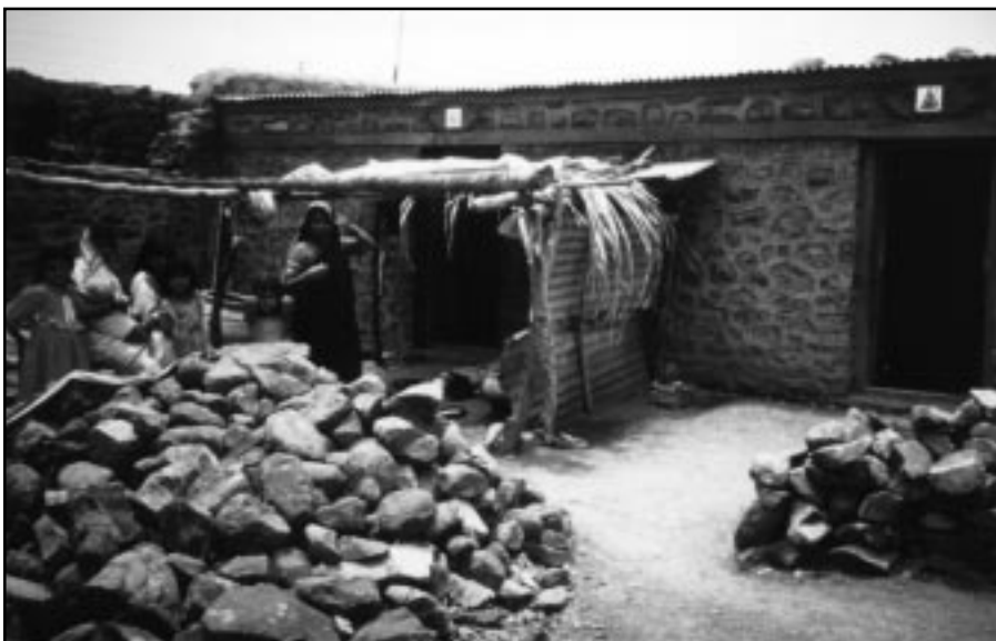
Figure 20 A stone masonry house reconstructed in an improved manner. The round stone boulders dismantled from the original house were not used for the construction.
