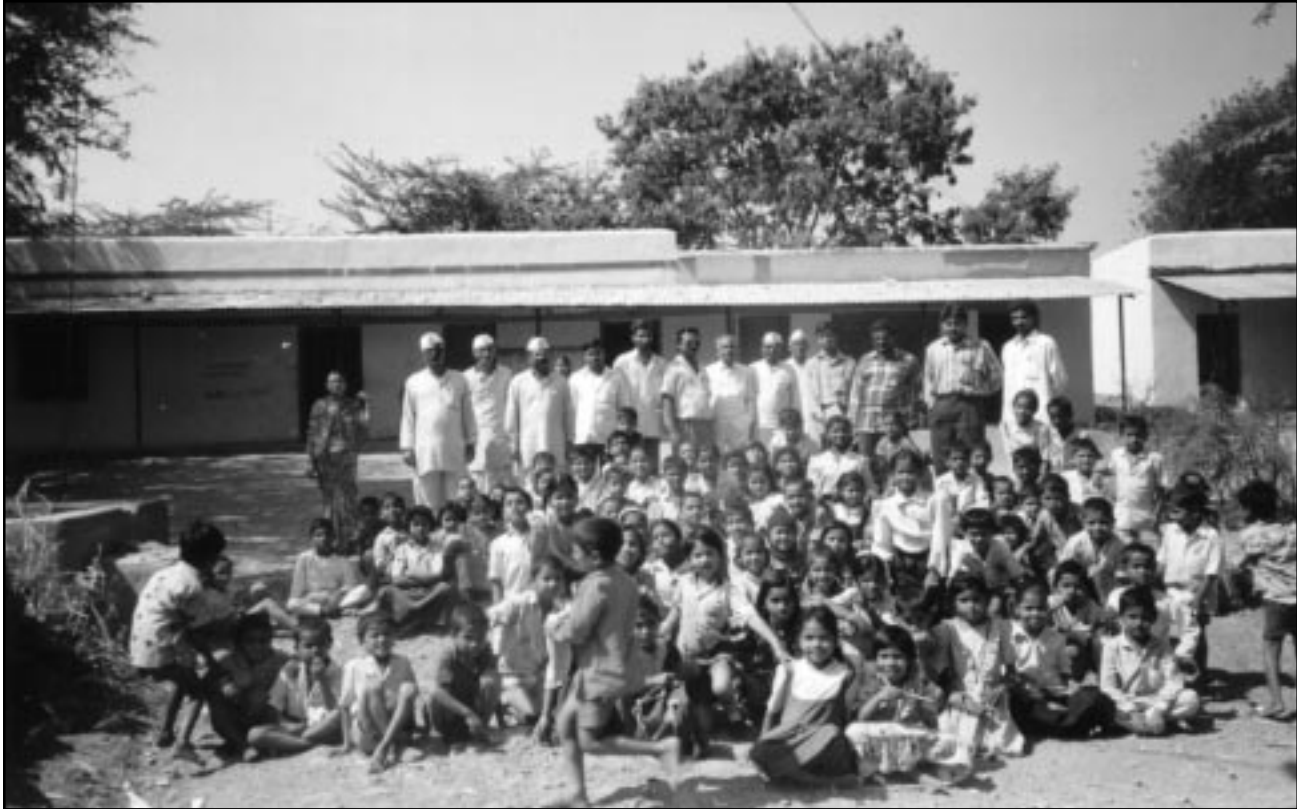
Figure 39 Students and teachers in front of a retrofitted elementary school building in the Latur district. The concrete bands are dark stripes near the top of the buildings.
