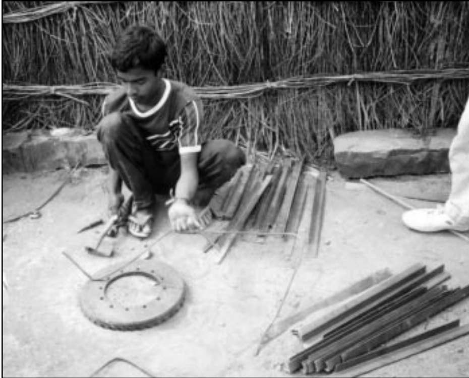
Figure 33 A village artisan working on fabrication of steel hoops for seismic bands and knee-bracings (rolled steel angles at the right).
