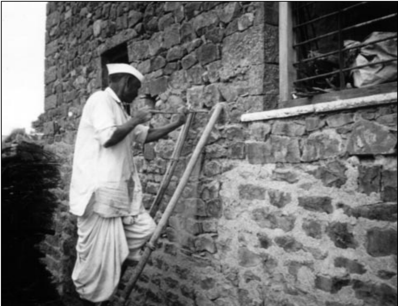
Figure 32 A village artisan preparing to install a through-stone. Here, he is removing a stone with a crowbar.
