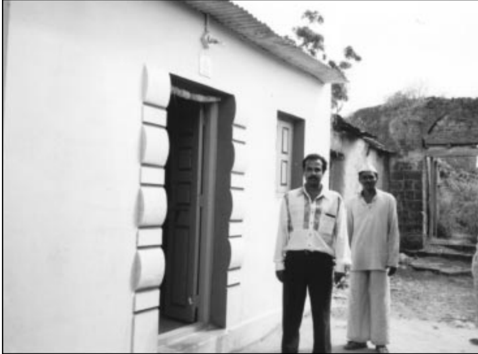
Figure 31 A Junior Engineer (in black trousers) with a beneficiary standing in front of a completed house in the repair and strengthening program.
