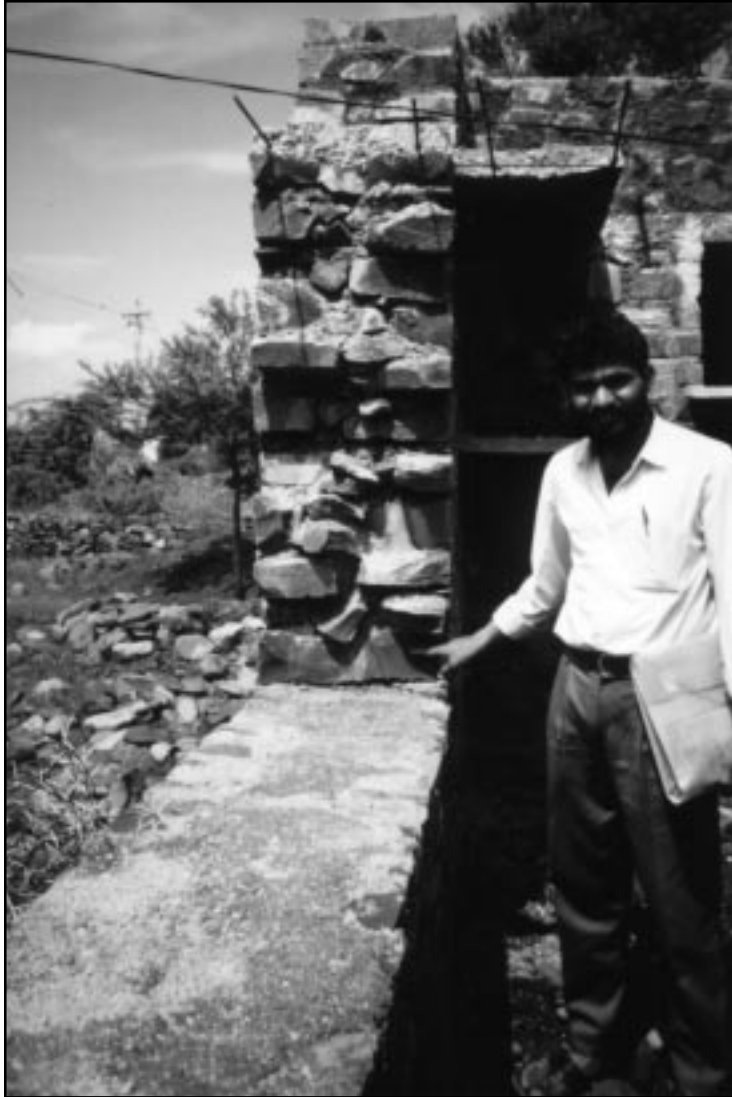
Figure 29 A GOM Junior Engineer inspecting a newly built stone wall and pointing out a through-stone.
