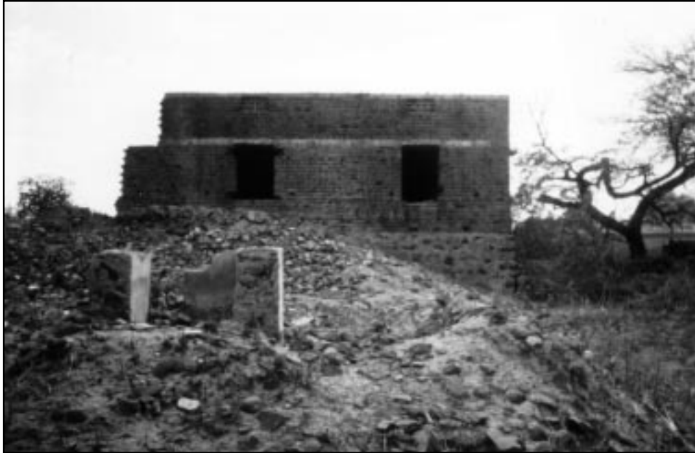
Figure 18 An unreinforced masonry building constructed to the higher standards and with a concrete lintel band survived the 1993 earthquake without any damage (Killari village, Latur district).
