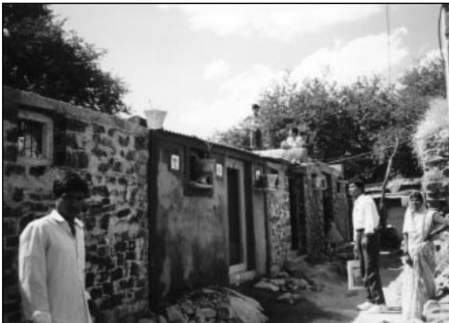
Figure 24 In some villages, stone masonry remained the most popular building material after the earthquake. Here a Junior Engineer is inspecting several new stone masonry houses.
